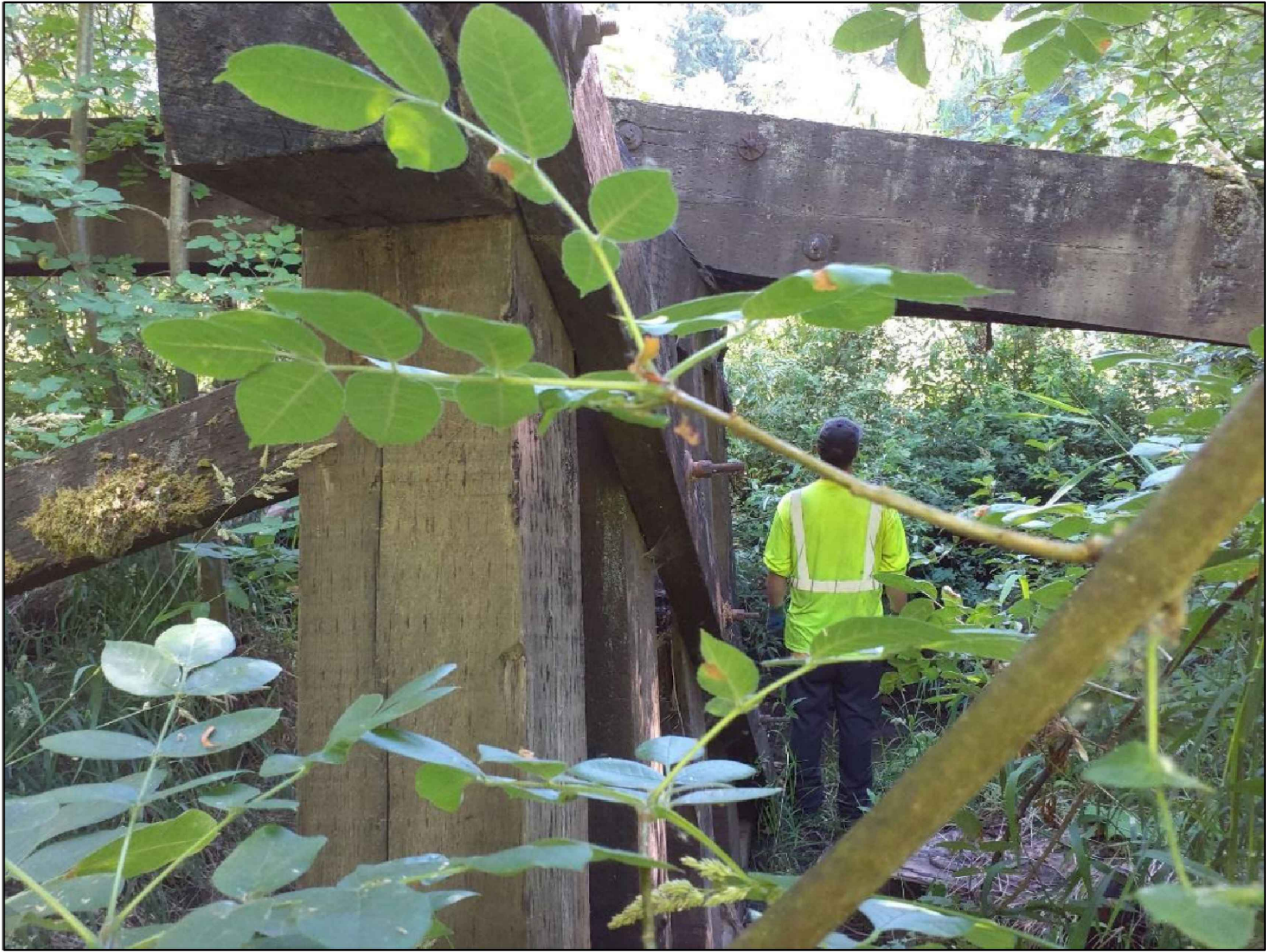
IMAGES OF THE TRESTLES TO BE REMOVED
