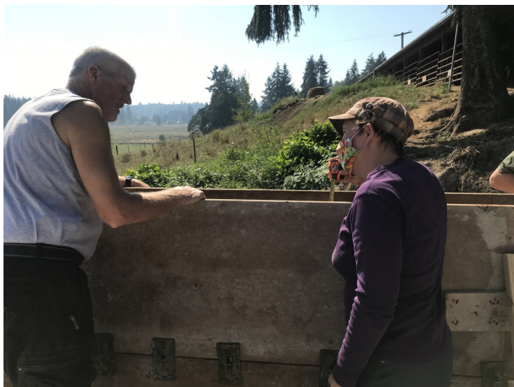
District Engineer, Katrinka Hibler, inspects the wall of a newly constructed waste storage facility with the landowner
